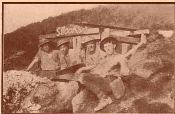
Building a "Spooks" (Battery Sigs.) Control Station, Bresle, France.
